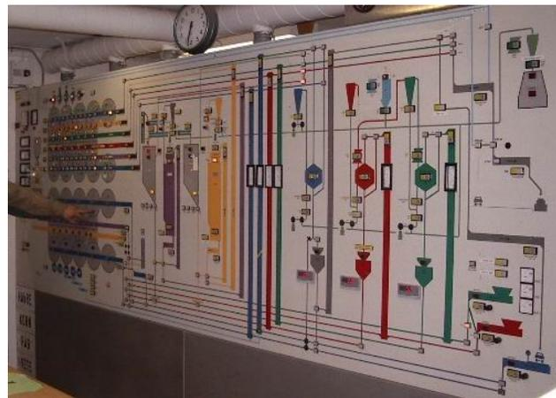
Figure 2. The electronic control panel, with integrated representations of the silos (upper left) and the machinery, through which the plant is operated.
