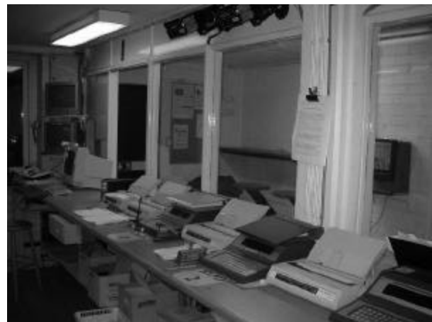
Figure 2. Above the desk, near the ceiling are three scales (black "boxes") used for monitoring grain transportation processes. On the desk lie printers (connected to the scales) and piles of documents.
